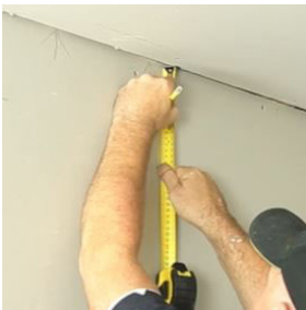
1. Marking Ceiling and Walls
