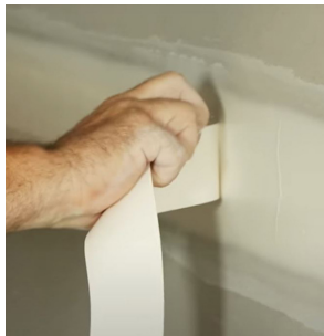
First Coat - Taping
