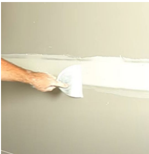
First Coat - Bedding compound
