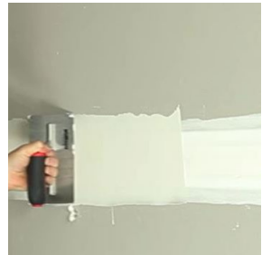
3. Apply Cornice adhesive
