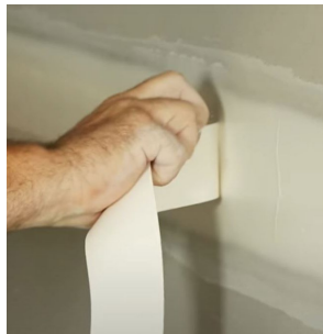
First Coat - Taping
